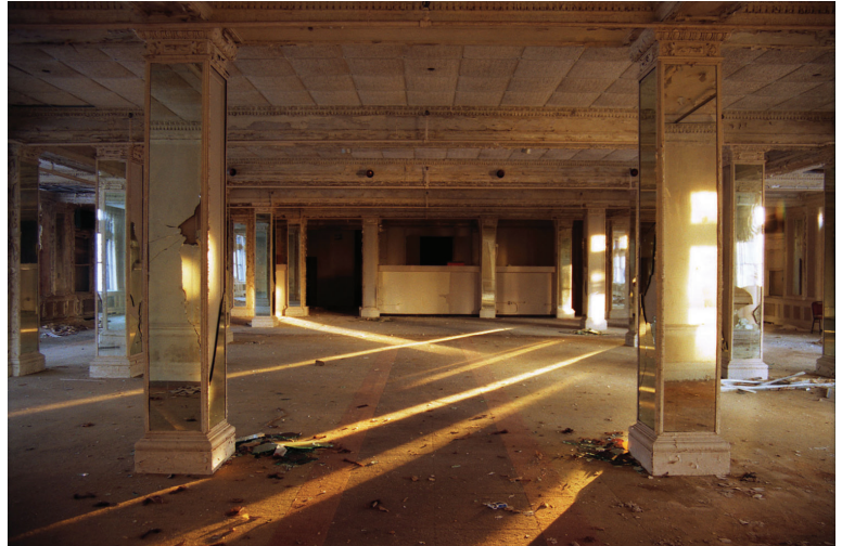
Robert Yasinsac - Briarcliff Lodge (Demolished), Briarcliff Manor, Westchester County, February 4, 2001
